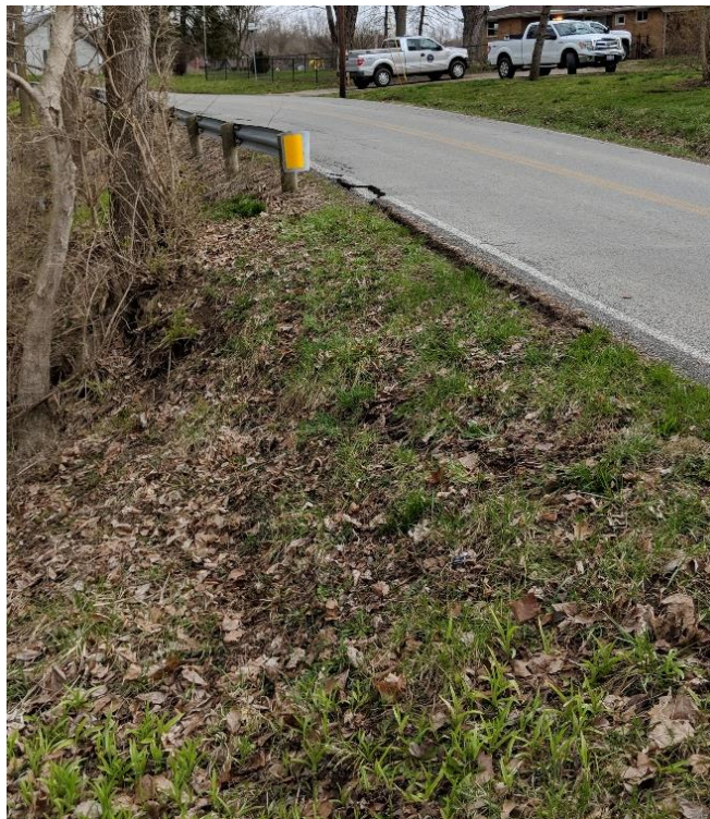
Photo 1: Site conditions observed on April 6, 2018
